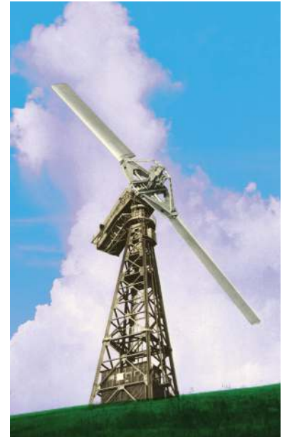
The Historic Smith-Putnam wind turbine in Castleton, Vermont 1941
