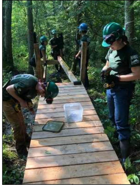
Figure 13: Marsh Trail Construction – Town of West Rutland
